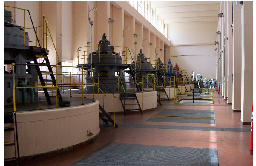
Figure 8.3 – Hydroelectric turbines at the Los Nihuiles Power Station in Argentina
