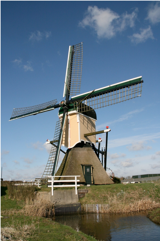
Photo by Quistnix at nl.wikipedia 2009 Figure 8.6 – A windmill in the Netherlands used to drain wetlands
